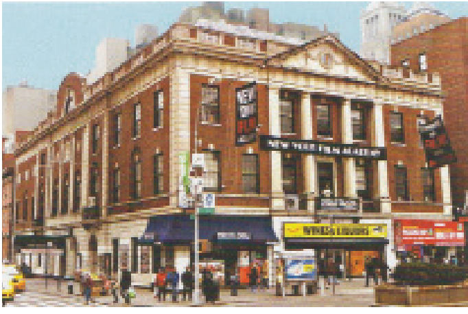
Former Tammany Hall
