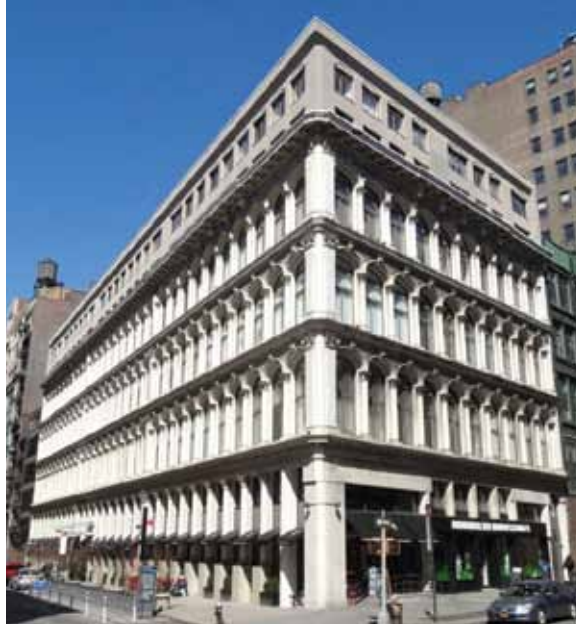
A | 801 BROADWAY (1868) AT EAST 11TH STREET FORMER JAMES MCCREERY DRY GOODS STORE
